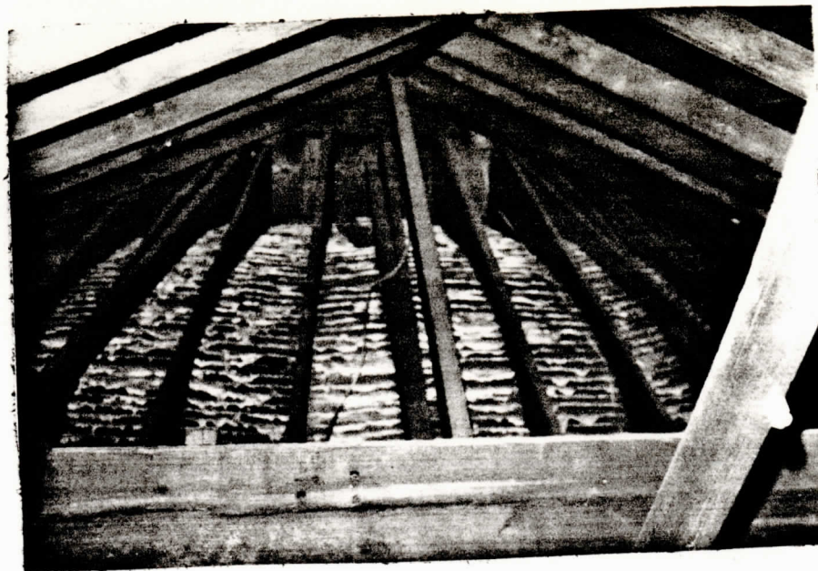
Figure 9. Detail of dome construction
